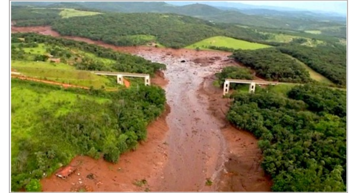
Tailings Dam Failures
